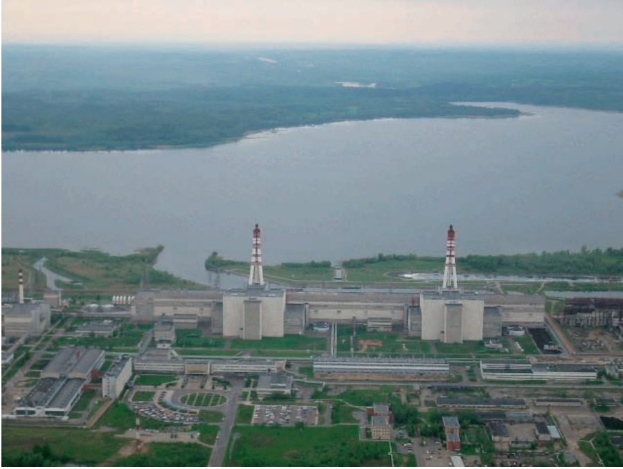
FIG. III-2. View over Ignalina NPP.
