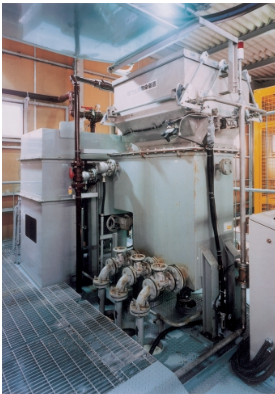
FIG. 5. Strong chemical decontamination apparatus, Nuclear Power Engineering Corporation, Japan.
