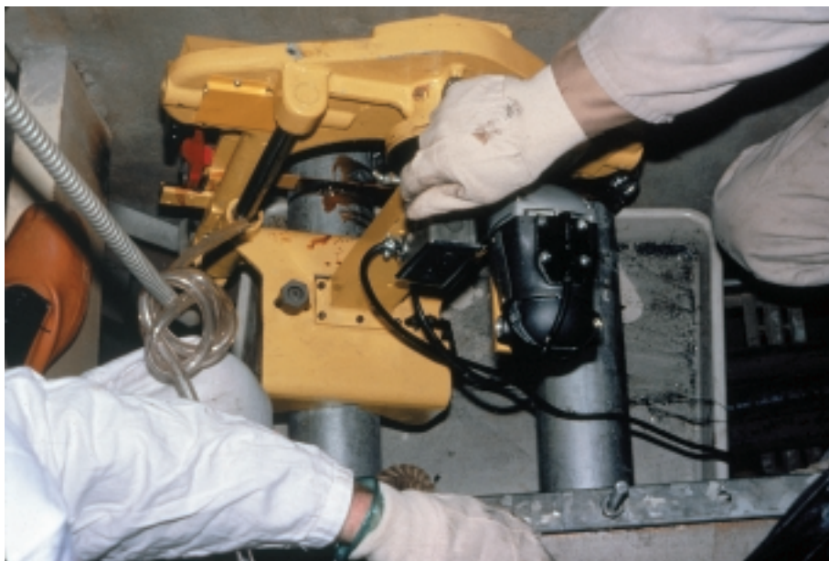
FIG. 19. Guillotine saw in use at Gentilly-1, Canada.
