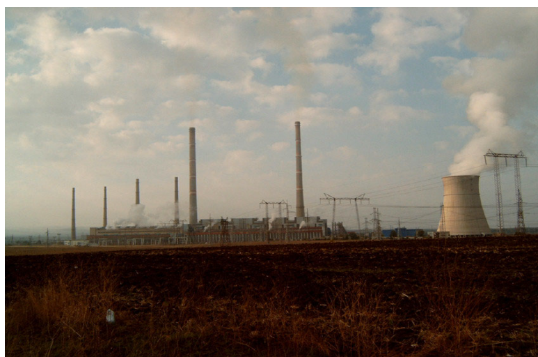
FIG. 5. General View of Maritsa – East 2 TPP PLC.
