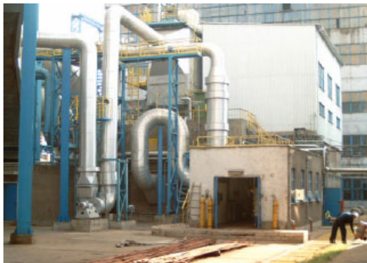
FIG. 1. Electron beam plant
