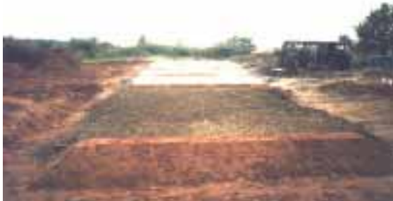
Preparation of the lime-based barriers
