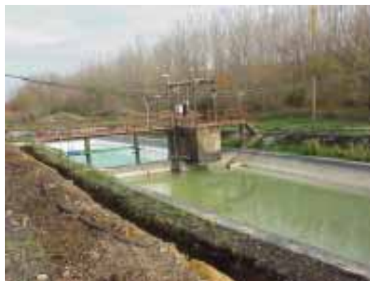
Basins for extracted groundwater and treated water
