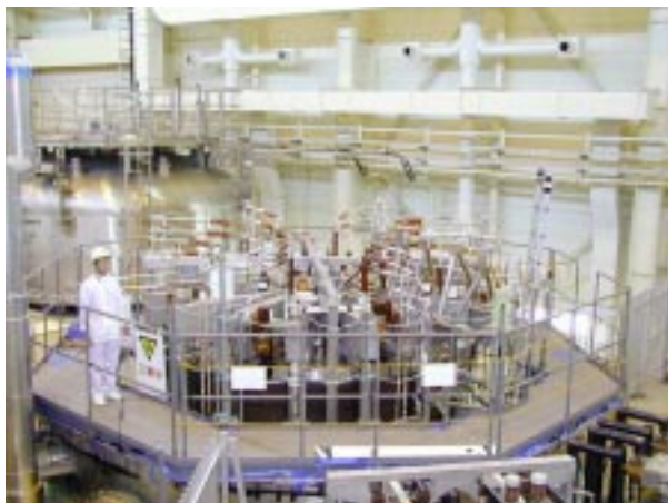
FIG. 8. CS model coil and CS insert installed in the vacuum chamber at the test facility in JAERI Naka. The preload structure (upper beams and tension rods), helium pipes and tops of the coils are visible.
