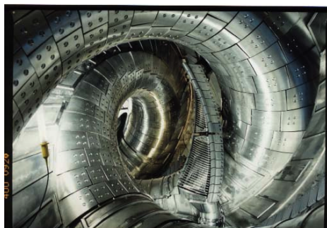
Fig.1 The ICRF antenna used in the experiment. The antenna is located in the toroidal section where the cross section is vertically elongated.
