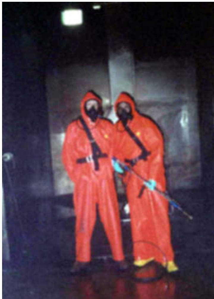
FIG. 35. Workers with personal protective equipment and HPWJ lance (courtesy: Atomic Energy Commission of Syria).
