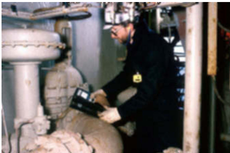
FIG. 25. Monitoring the outside of plant and equipment using a dose rate meter (courtesy: National Radiological Protection Board, UK).
