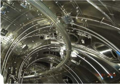
*FIG. 2. In-vessel cryo-pump after installation*
