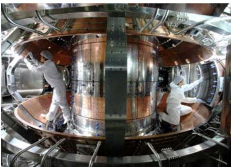
*FIG. 4. Passive stabilizer under installation in the vacuum vessel*
