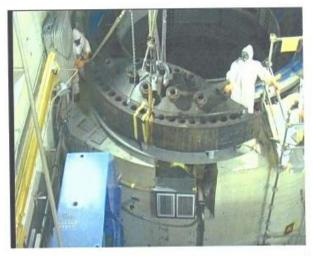
Fig. 13: First segment of RPV closure head onto its temporary position on the biologic
