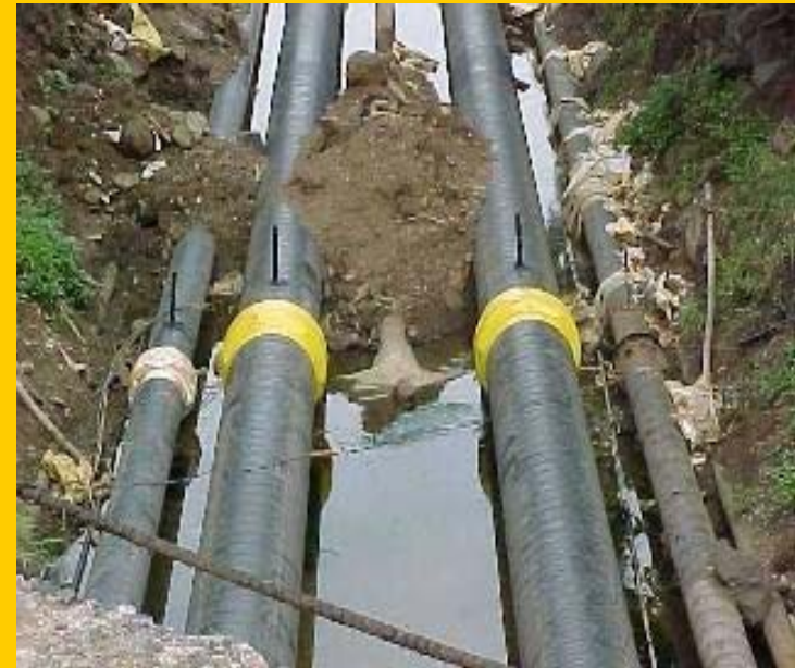
Reconditioning of underground piping in primary cooling system of Cirus
