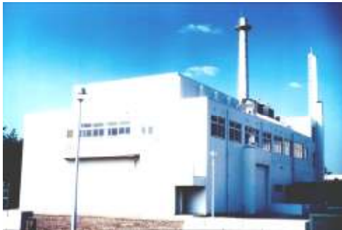
Actinide research facility Oarai branch, Tohoku Uni.
