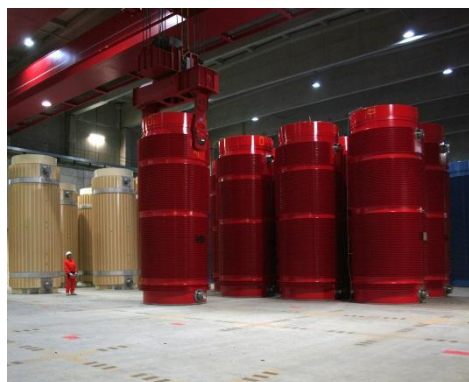
Transport and storage casks in the Transport Cask Storage Facility Gorleben (Photo: GNS)
