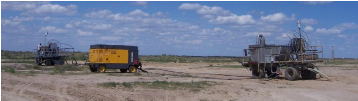
Wells Treating Portable Equipment
