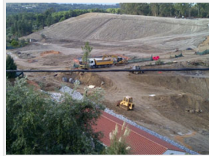
The Cunha Baixa uranium mine site, Portugal, under remediation by EDM
