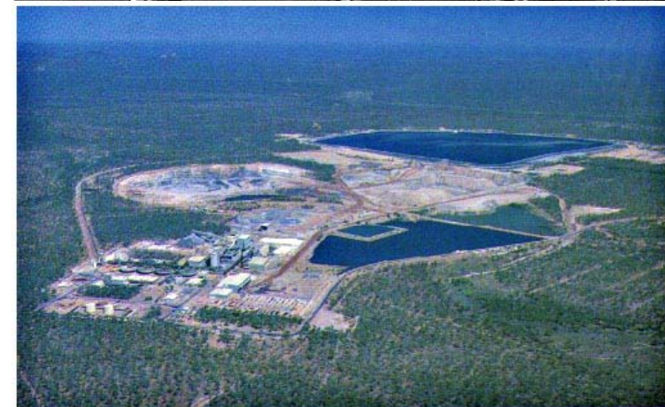
Aerial view of Ranger Mine and Plant
