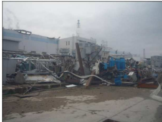
Unit 3 Sea Pump Area
