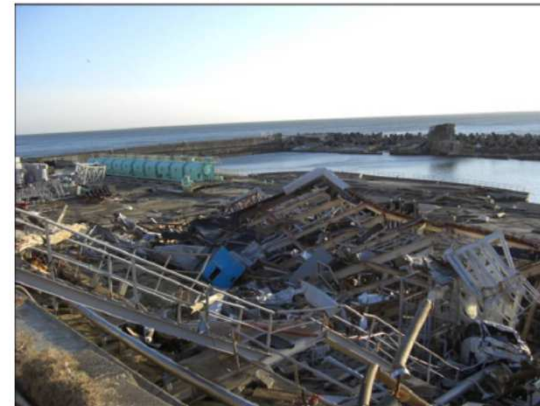
Unit 5,6 Intake Screen Area
