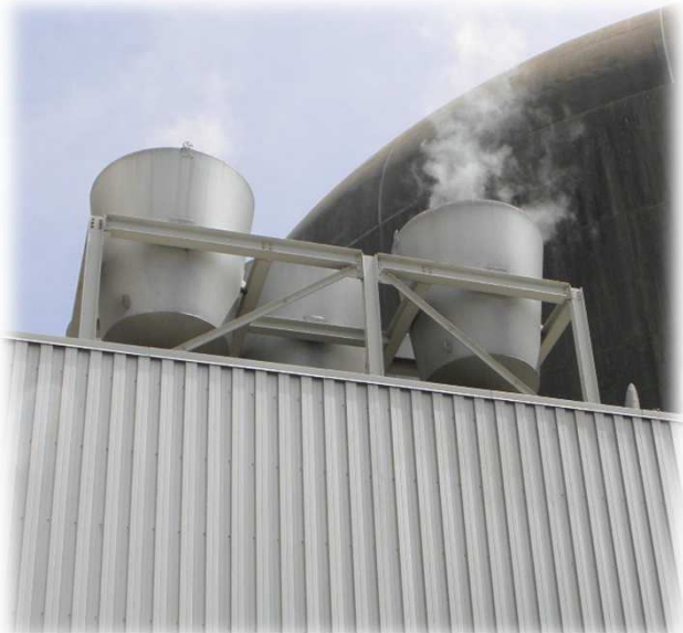
Steam Reject Valves to depressurize Steam Generators
