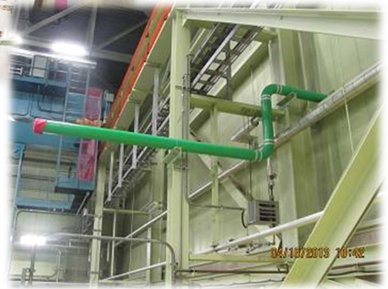
EME Water Supply piping to IFB
