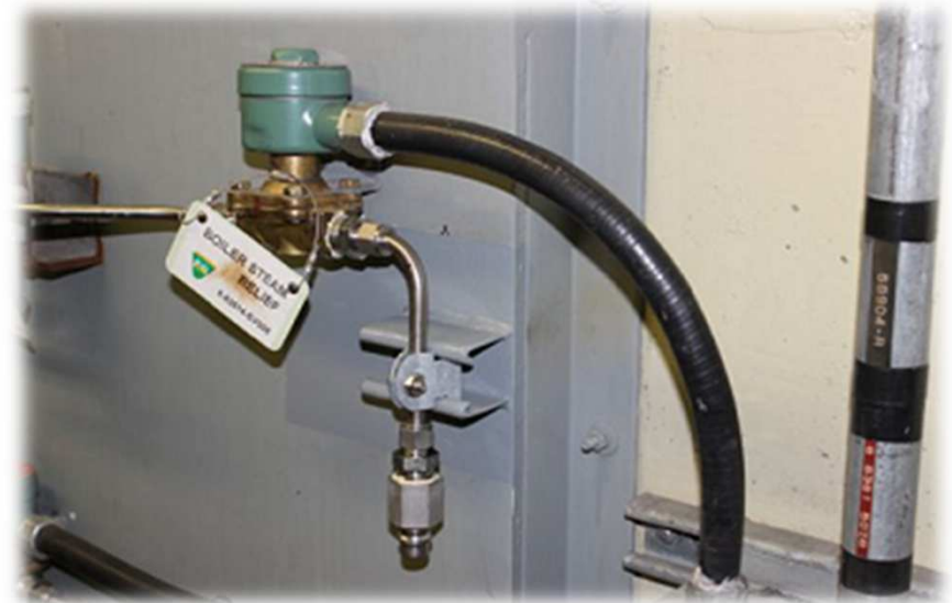
Additional Air supply to hold Steam Reject Valves open
