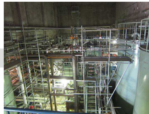
Construction in RW building
