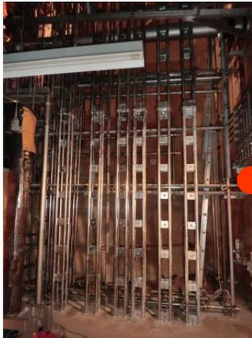
Photo② Steel posts installed condition (Before concrete placement)
