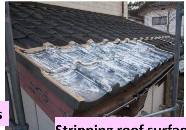
Stripping roof surfaces
