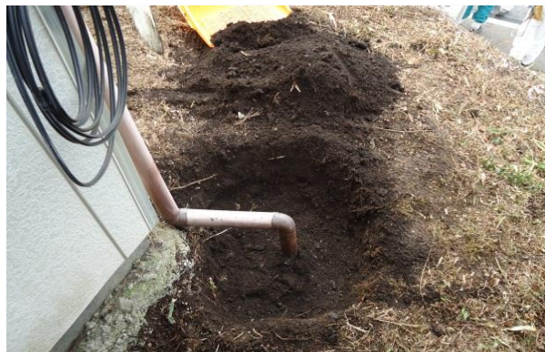
Removing drainage hotspots
