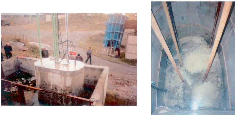
FIG. 9. Mock-up of grouted IRT reactor in Georgia.
