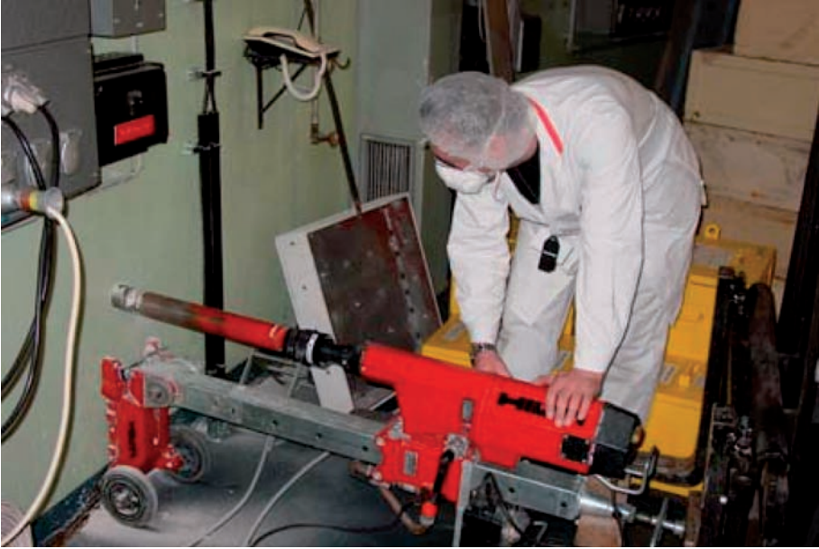
FIG. 8. Core drilling tool at the Astra research reactor.
