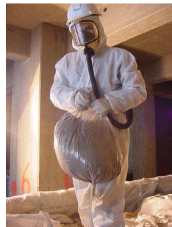
FIG. 6. Outfit for personal protection during dismantling.
