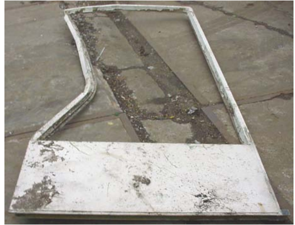
FIG. 4. A door insulated with slag wool.
