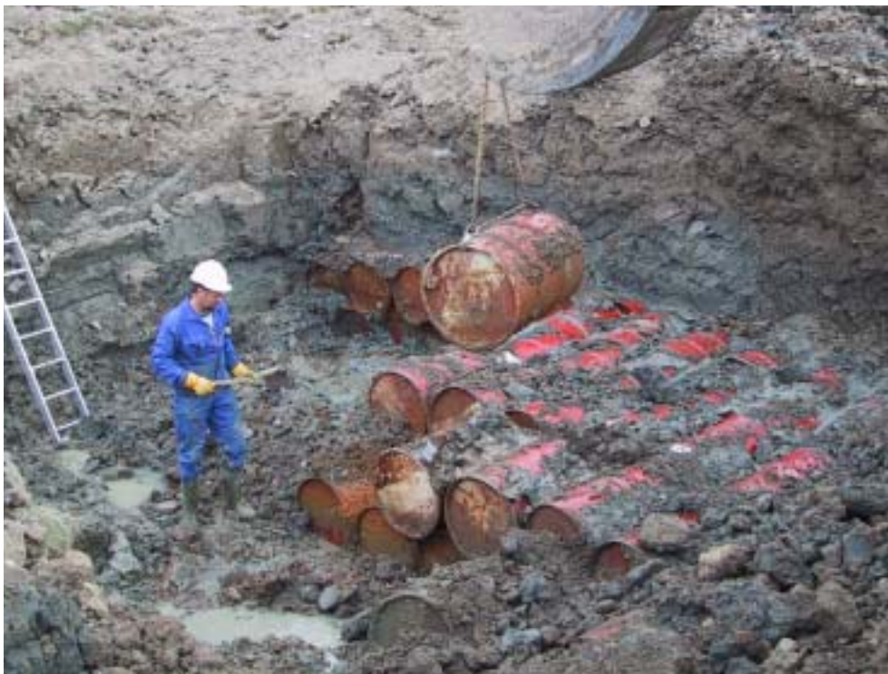
FIG. 2.1 Retrieval of the waste drums.
