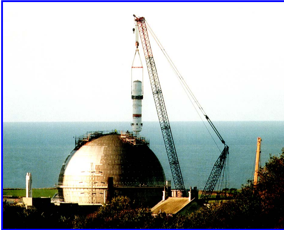
Figure 5-2: Removal of Heat Exchanger from the Windscale AGR
