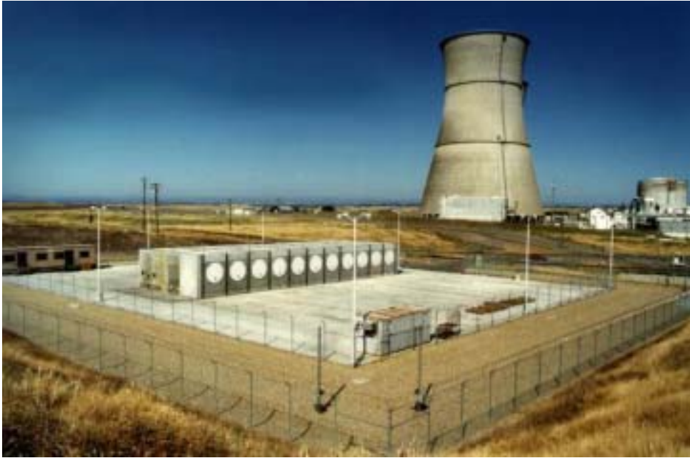
FIG. 7. Typical horizontal storage module configuration.
