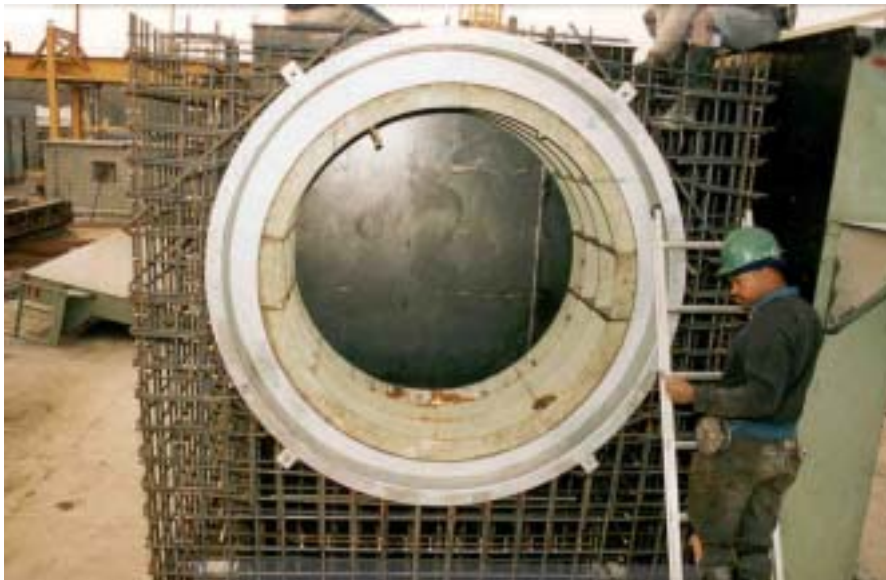
FIG. 3. HSM fabrication.
