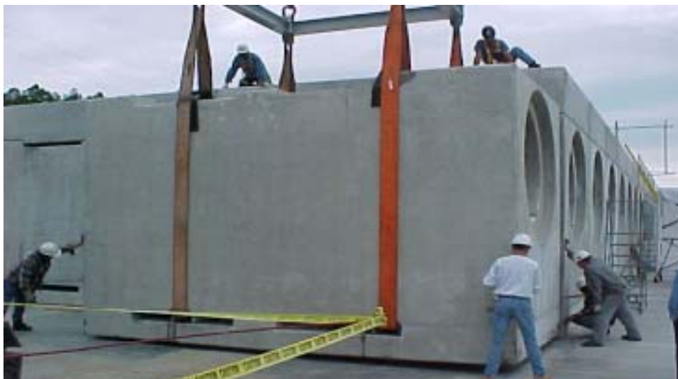
FIG. 4. HSM Installation at an ISFSI site.
