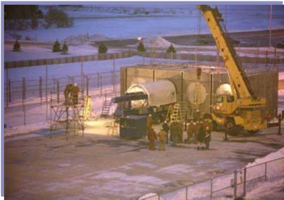
FIG. 8. Placing the canister in the HSM.
