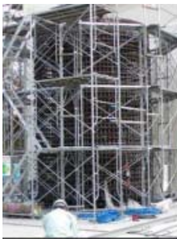
[Arrangement of reinforced bar]
