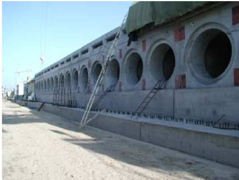
FIG. 8. The alley of FRAMATOME's Chernobyl NUHOMS ® .
