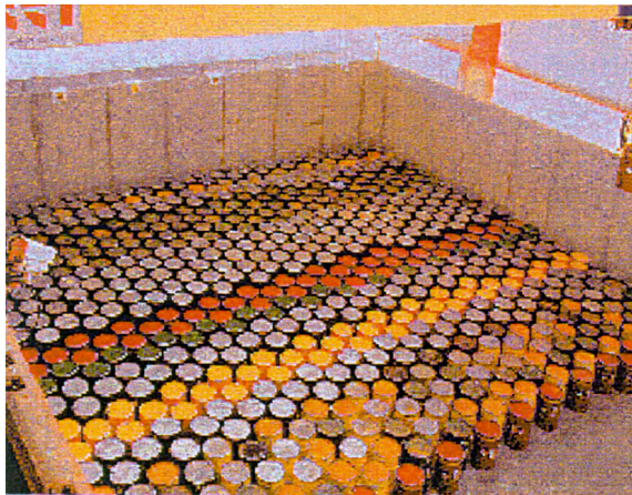
FIG. 4. Waste package emplacement.
