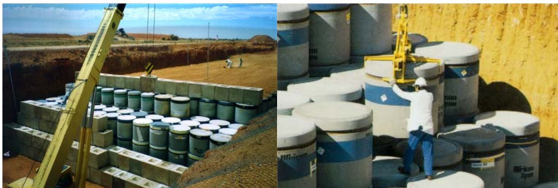
FIG. 5b. National Radioactive Waste Repository Vaalputs Intermediate-level Radioactive Waste Disposal
