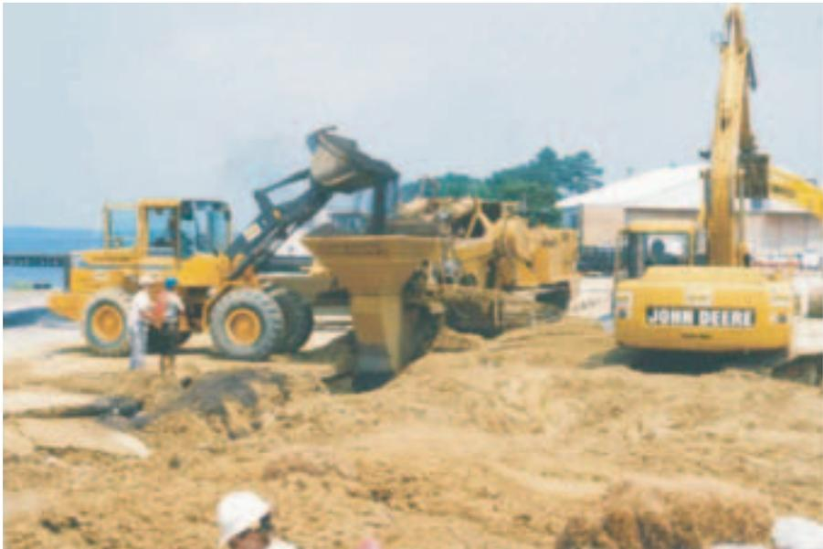
*FIG. 7. (a) Continuous trenching machine used to install the 46 m long, 7.3 m deep and 0.6 m wide granular iron permeable reactive barrier; (b) simultaneous excavation and replacement of aquifer material with granular iron as the horizontal trencher advances [193].*
