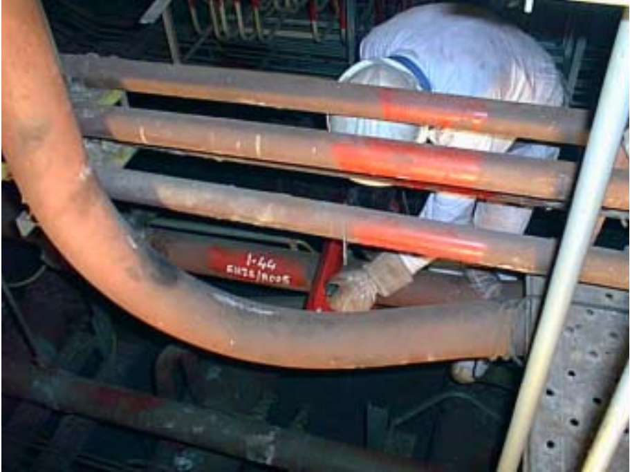
FIG. I-28. Vandellós NPP unit 1, cutting steam generator pipes.
