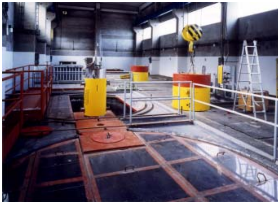
FIG. I-1. Storage facility for spent fuel and high level waste (HLW) with container for transporting LVR-15 spent fuel.
