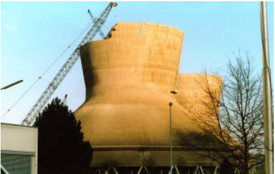
FIG. I-11. Demolition of the cooling towers of the Würgassen NPP.
