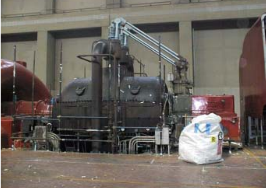
FIG. I-13. Asbestos removal at the Trino NPP.
