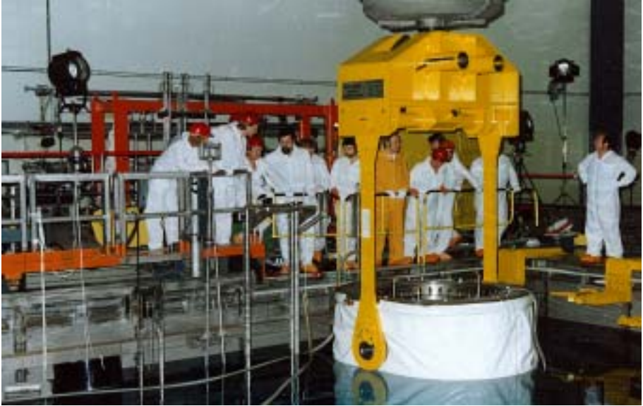
FIG. I-10. Removal of irradiated fuel elements from the core of the Würgassen NPP.
