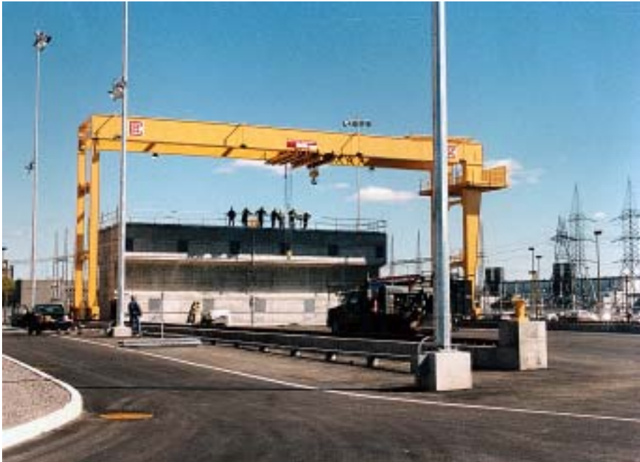
FIG. 10. CANSTOR™ concrete module for interim dry storage of CANDU type spent fuel, Gentilly-2 NPP, Canada.
