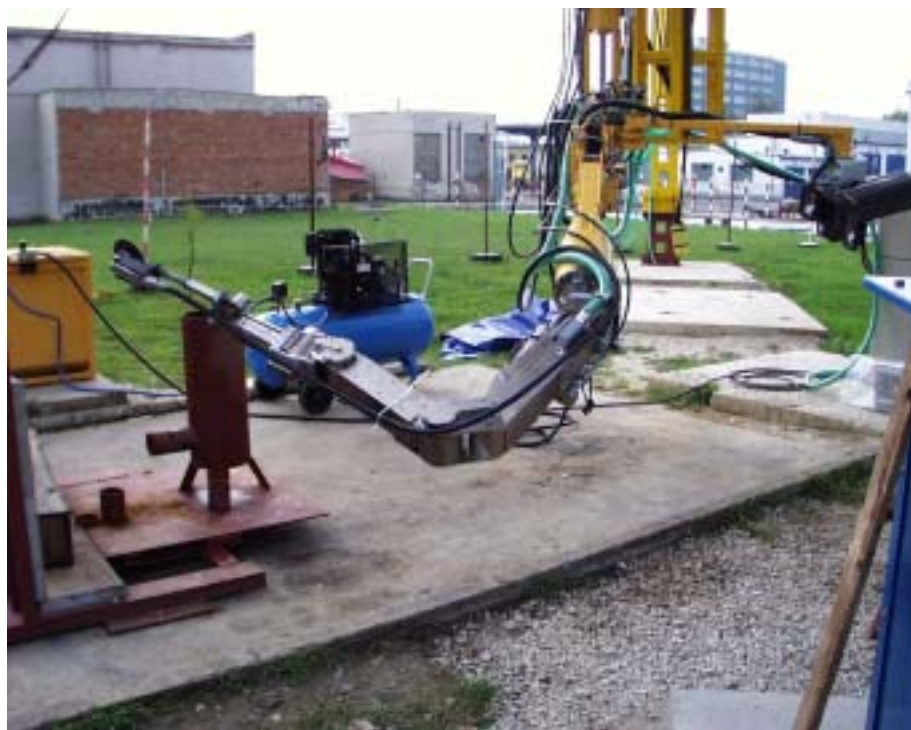
FIG. 6. Mock-up test of the manipulator at the A-1 reactor decommissioning project in Bohuniče, Slovakia.
