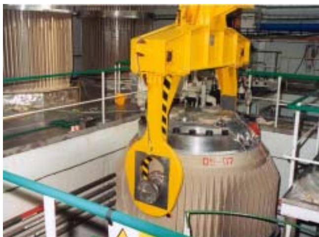
FIG. I-26. Transport cask for transferring spent fuel from the V-1 and V-2 NPPs to the interim spent fuel storage facility.
