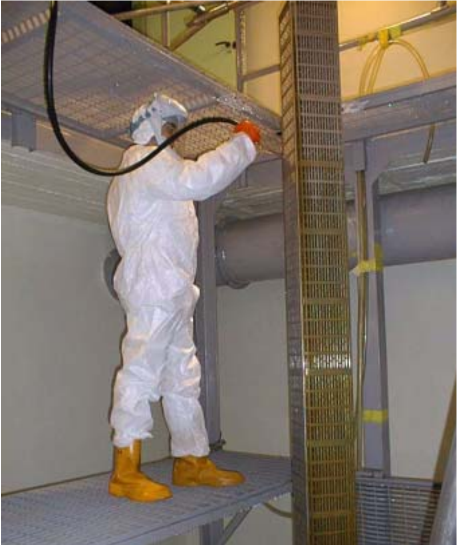
FIG. I-17. Fresh fuel decontamination for shipping from the Trino NPP.
