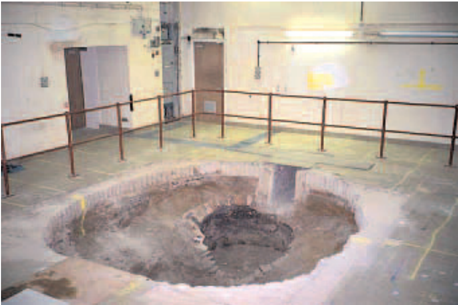
FIG. II-5. Site appearance after the completion of the decommissioning.
