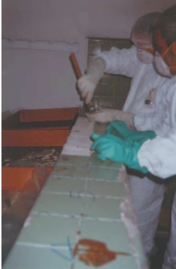
FIG. I.B-4. The contaminated tiles being removed.
