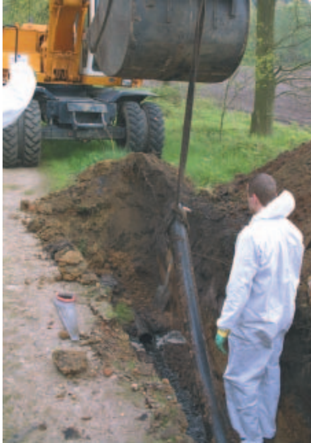
FIG. I.A–5. Excavation of the pipe.
