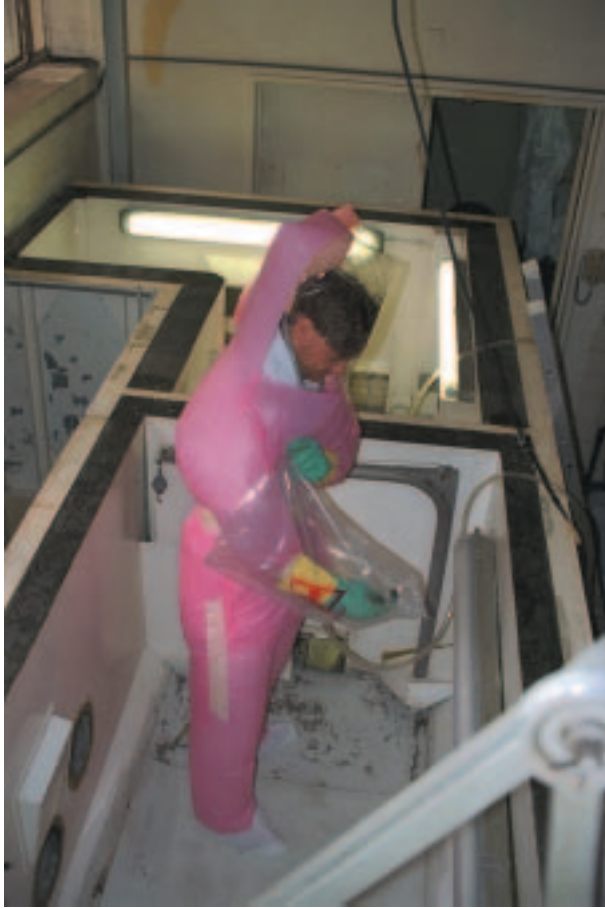
FIG. I.A-4. Protective clothes worn during the dismantling of a hot cell.
