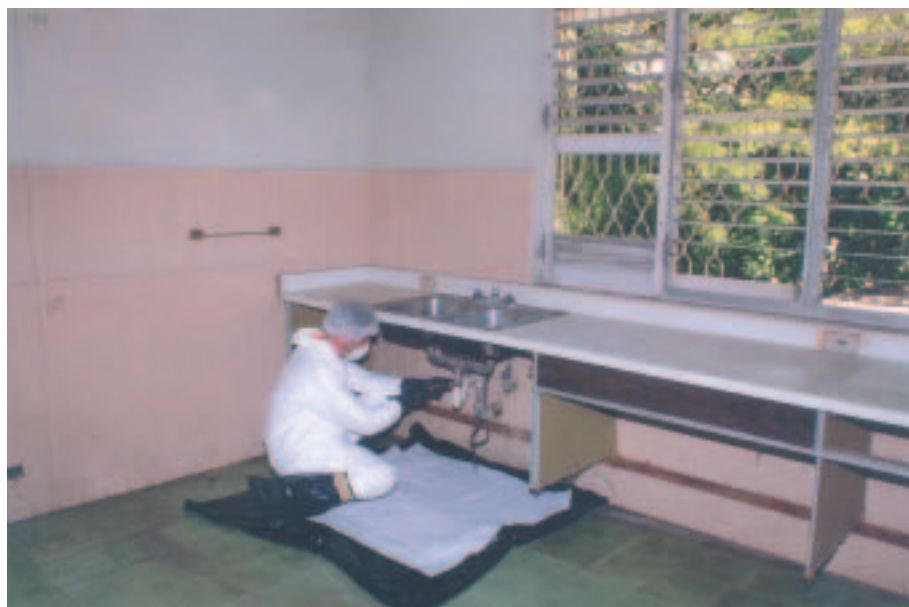
FIG. I.D–2. Patient room IV. Decontamination activities: dismantling the sink and looking for the sealed source.
