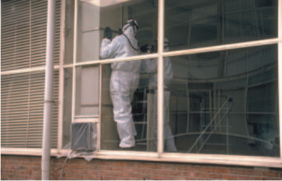
FIG. I.A-2. Dismantling ventilation pipes.
