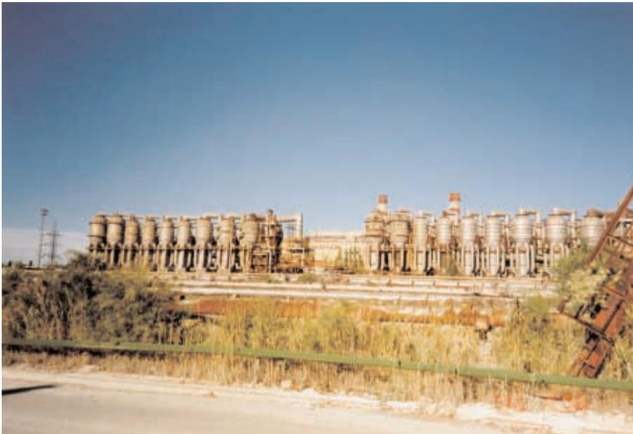
*FIG. 5.7. Evaporators for the nuclear desalination plant (LMFBR–MED) at Aktau, Kazakhstan.*
