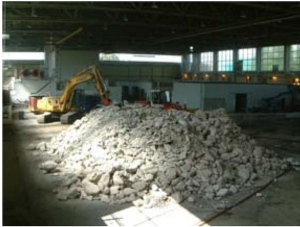
*FIG. 8. Concrete prior to crushing.*
