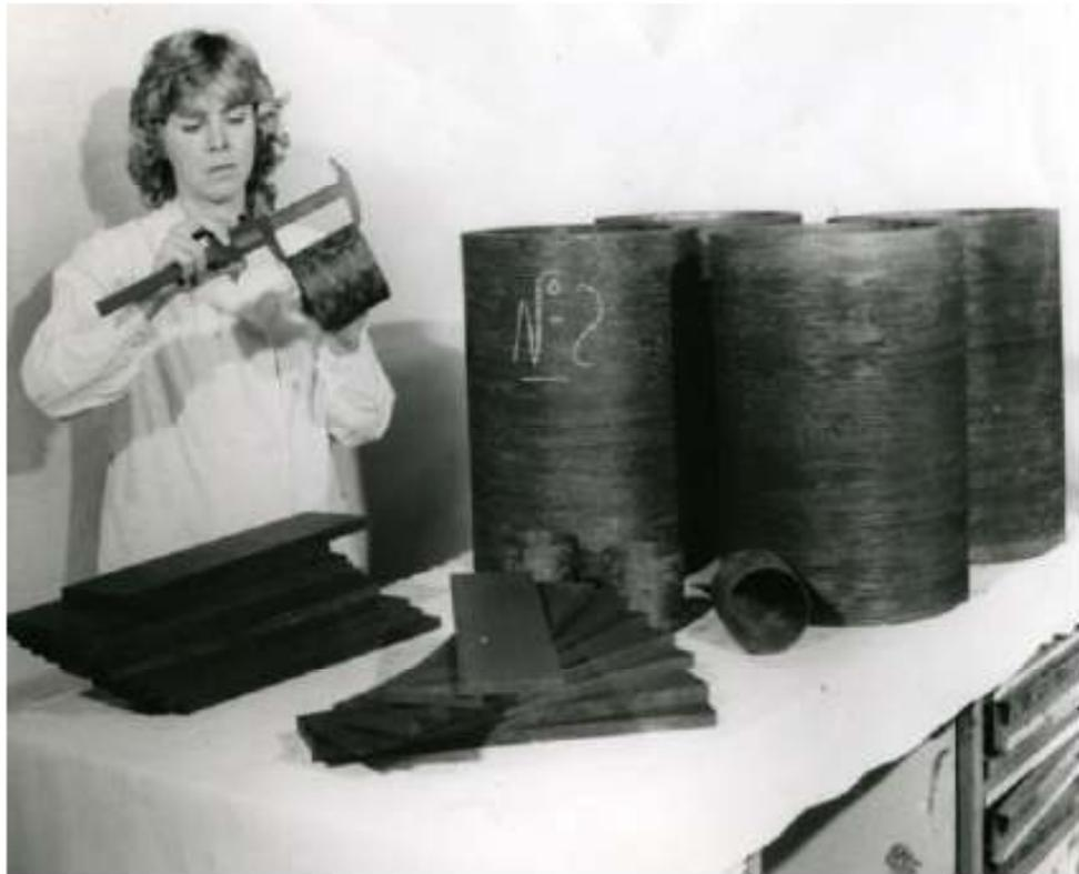
Fig.9a. Appearance of products and structures made of carbon-carbon composites: plates and crucibles for metal melting.
