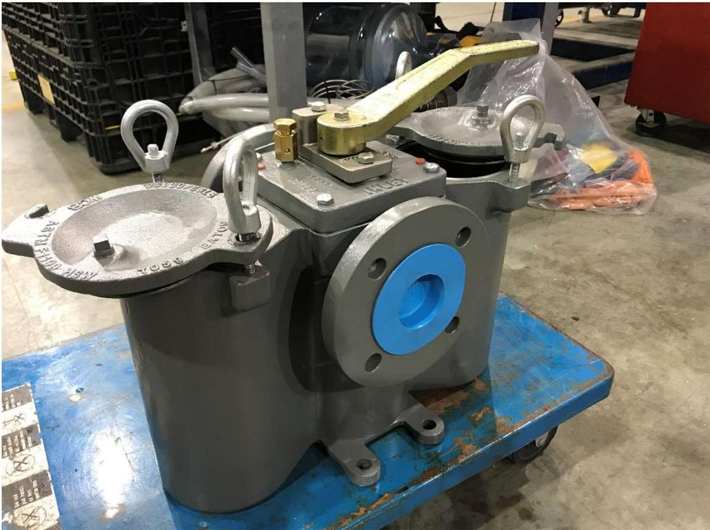
FIG. 16. Photo of duplex strainer (Courtesy of Kinectrics).
