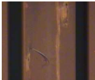
Wire sticking out of fuel rod – later removed with a plier tool – very small through-wall perforation (with bubbles present).
