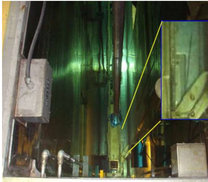
FIG. 12. The broken fuel rod of fuel assembly found in the fuel transfer channel.
