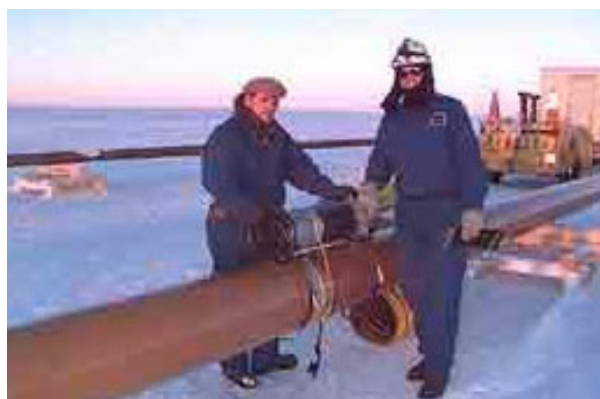
FIG. 18. Radiography testing inspection of a pipe welds.
