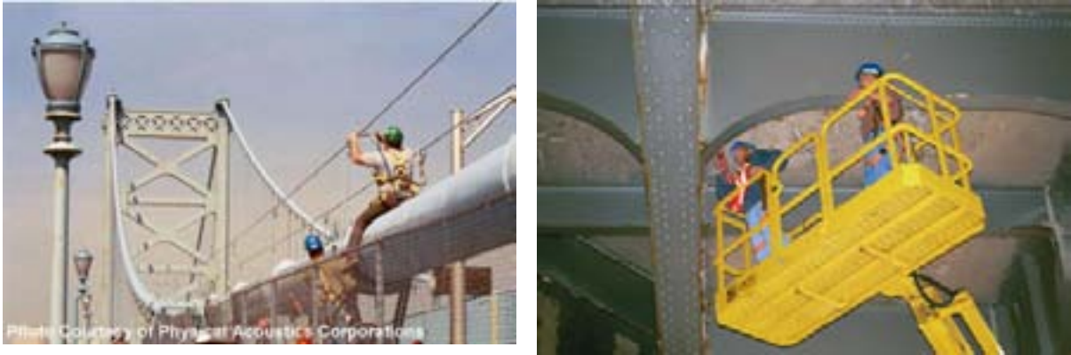
FIG. 22. Inspection of bridges.
