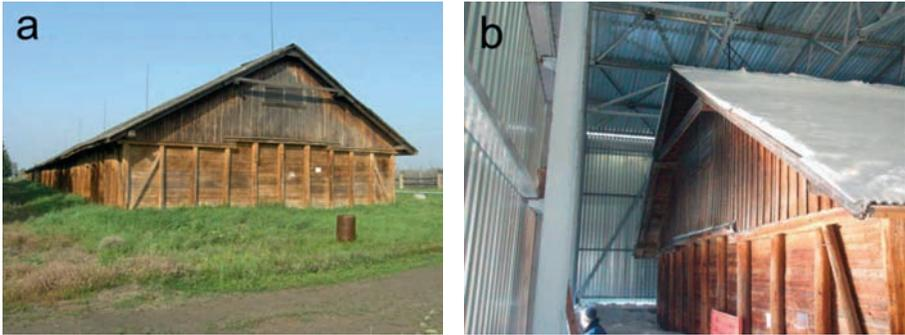
FIG. 1. One of the former granaries of the monazite storage facility before and after the repair work.
