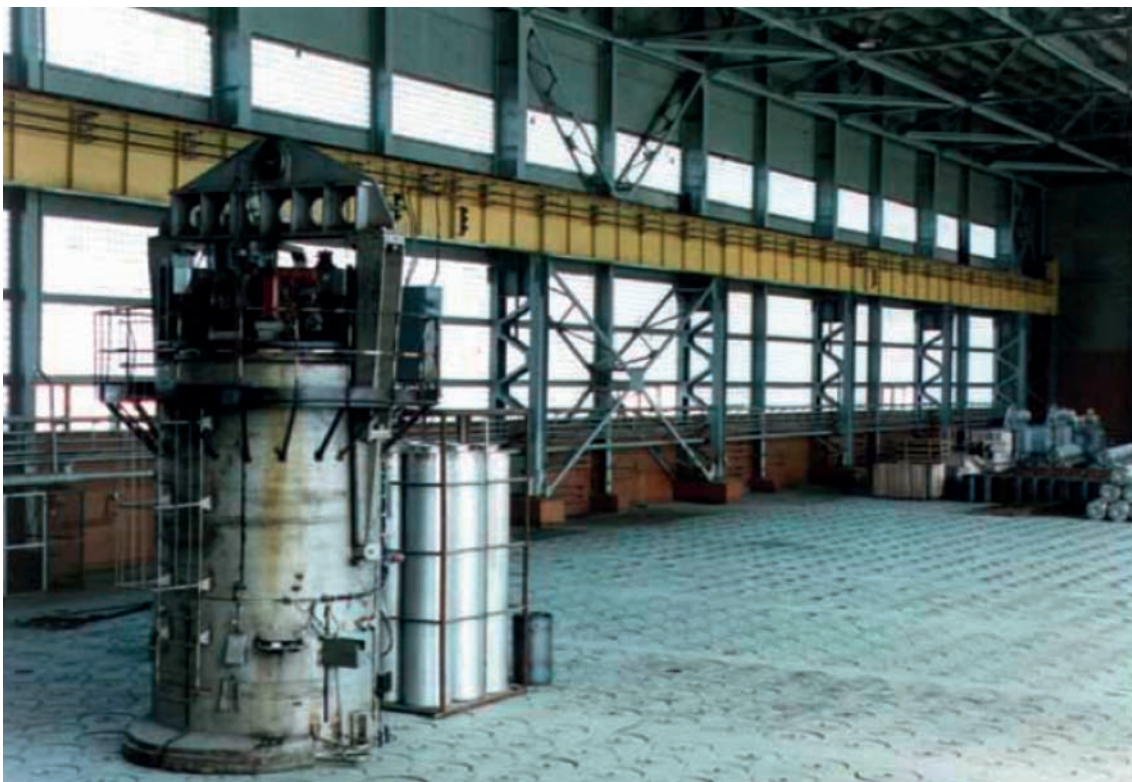
FIG. 15. Storage facility for vitrified waste at MAYAK.
