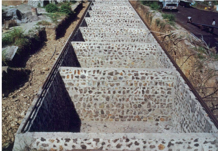
FIG. A-12. Stone lined earth trenches.
