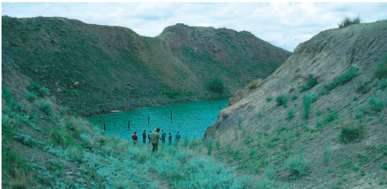
FIG. 4. Lake Tel'kem-2, which resulted from the fourth and last cratering nuclear explosion. The test was carried out using three nuclear devices, each the equivalent of 240 t of TNT [1]. The photograph was taken during the IAEA mission in July 1994.
