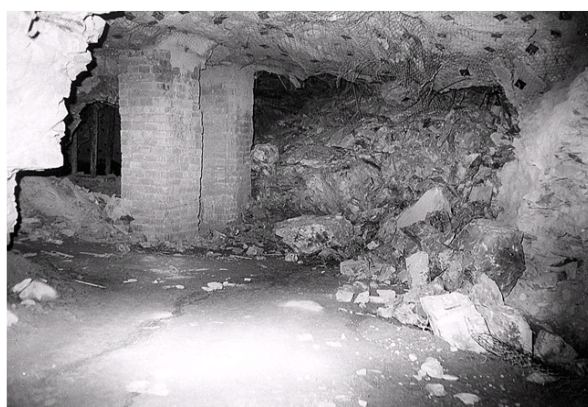
FIG.5. Mine stope roof demolition process (By Begus).
