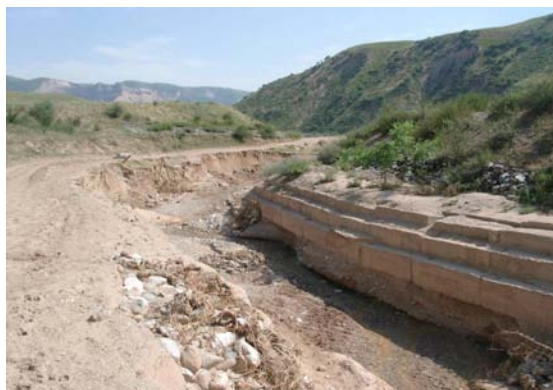
FIG.1. Fluvial erosion of the dam toe of tailings pond N° 2 and 13 in the valley of Aylampa Sai, a tributary of the Mailuu-Suu River.
