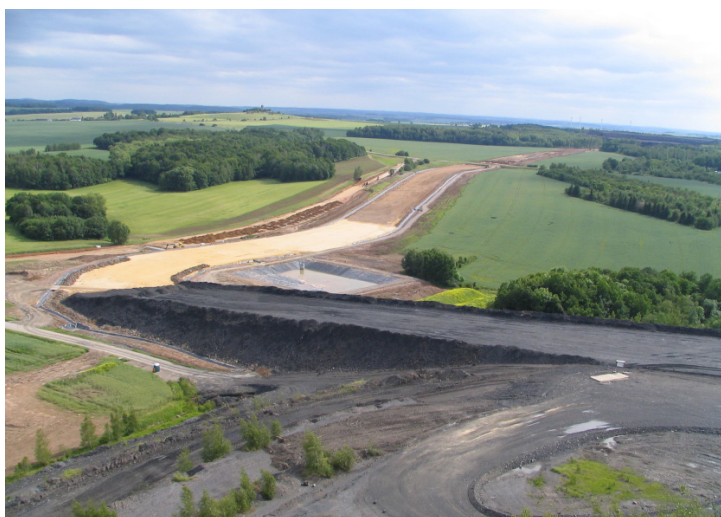
FIG.9. Construction of the transportation road from Halde Paitzdorf to the Lichtenberg open pit with waste rock. View from the dump towards the former Reust dump, which had already been relocated. June 2005.
