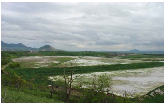
FIG.4. Covering of the tailings facility GMZ Lermontov using Phosphogypsum.
