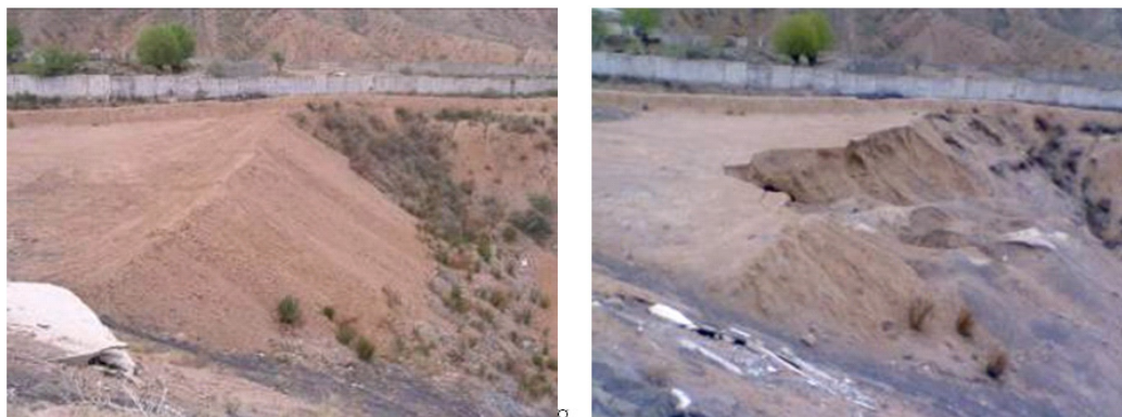
FIG. 7. The new containment dam (approximately 10 m high) and cover of the tailings (left) at the Kadji-Say facility built in 2005/6. The state of the new dam and cover damaged by water erosion in 2007 (right).
