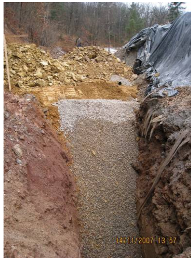
FIG.9. Excavation of the backside water drainage and fill with water conductivity materials to protect the mill tailing against the subsurface water inflow (Photo Likar).
