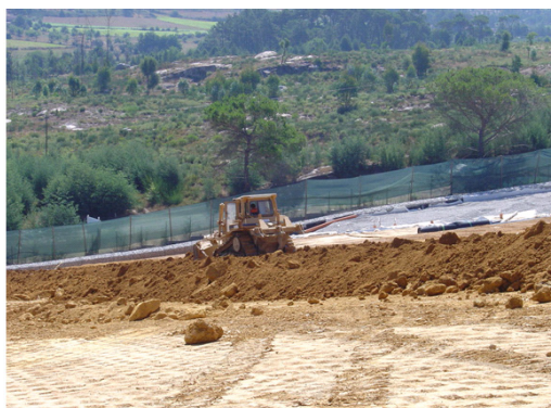
FIG. 5. Capping the main milling tailings at Urgeiriça (2007).
