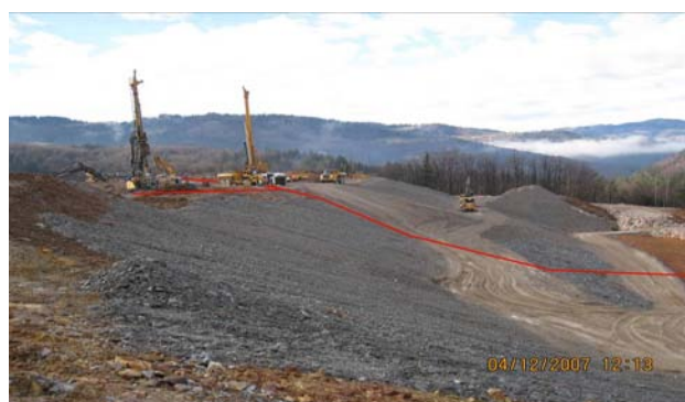
FIG.8. Excavation of the central drainage at the mill tailings (redline shows the course) (Photo Likar).
