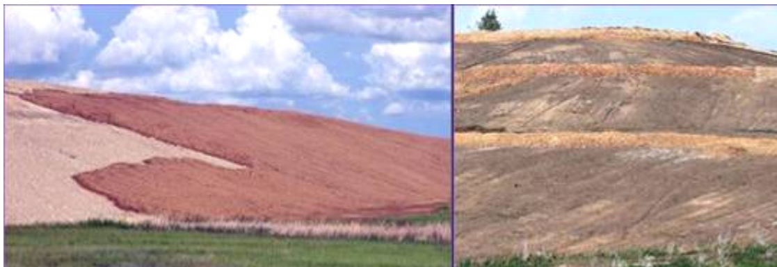
FIG. 8. Covering the remediated slopes of the waste rock pile on the site of the mine No. 9 in N. Kazakhstan.
