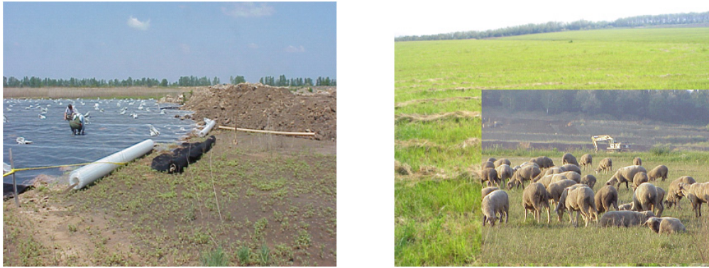
FIG. 8. Stabilization of the fine tailings zone on tailings pond and view on the remediated and revegetated tailings pile.
