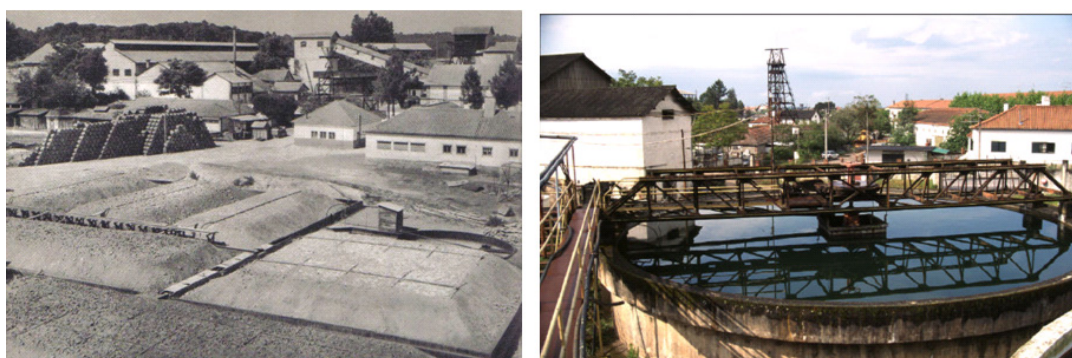
FIG.3. Uranium static heap leaching and dynamic uranium ore leaching tank facilities at Urgeiriça.
