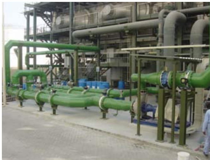
FIG. 24 Integrated upgrading temperature blending system at Layyah
