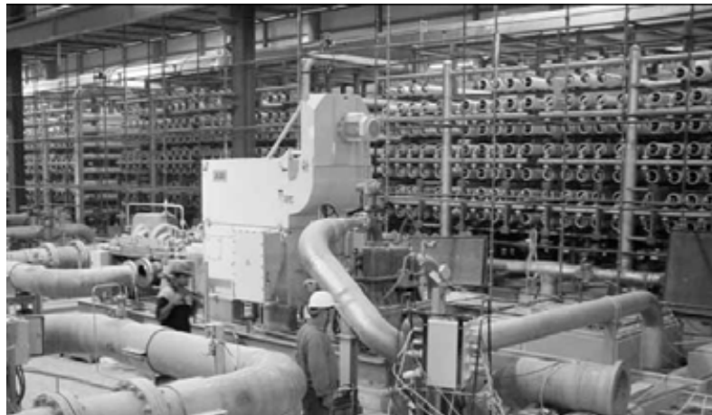
FIG. 18. Fujairah plant SWRO racks and feed pump/ER turbine
