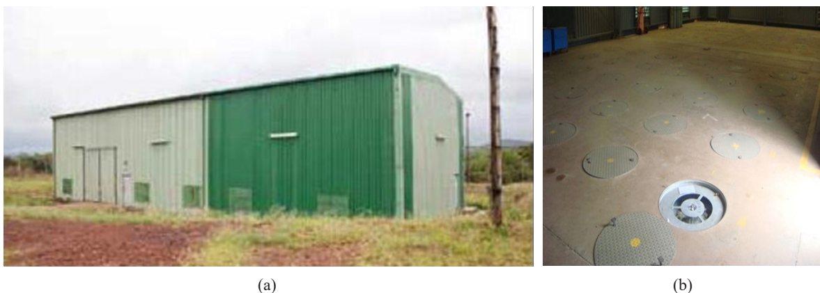
FIG. I-17. The Thabana Pipe Store dry storage facility: (a) exterior and (b) interior, showing an open pipe (courtesy of Necsa).
