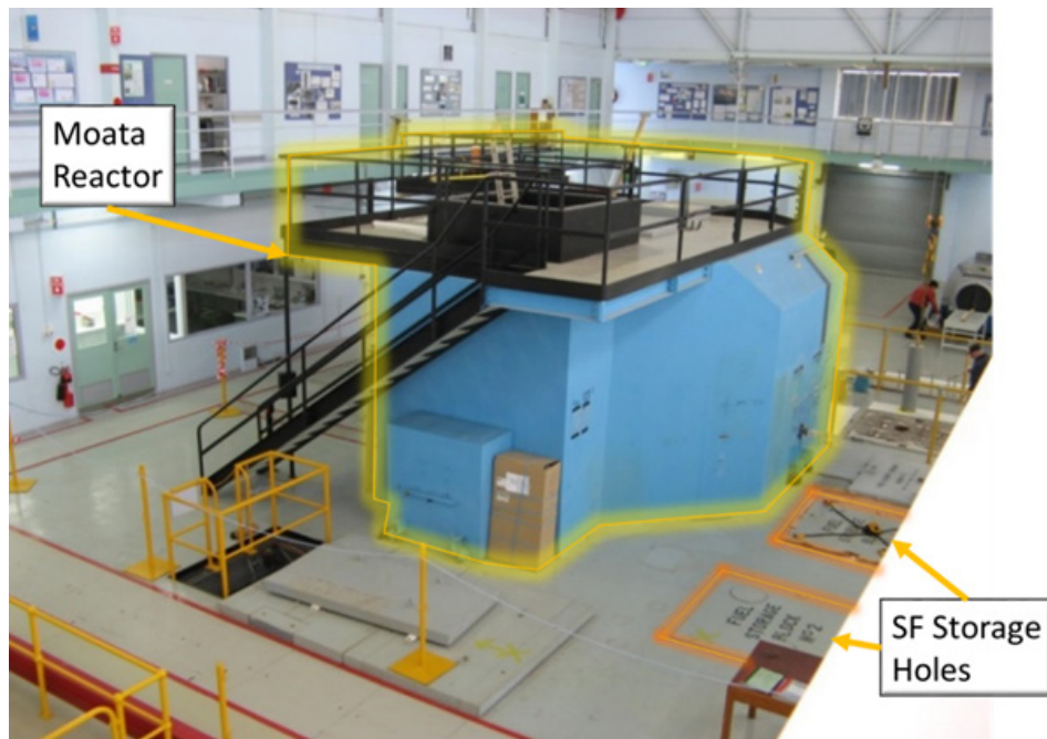
FIG. 9. The Moata fuel storage holes are visible on lower right hand side (courtesy of ANSTO).
