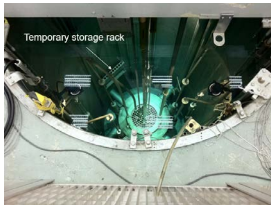
FIG. I-13. View inside the reactor pool showing the storage rack (courtesy of Malaysian Nuclear Agency).
