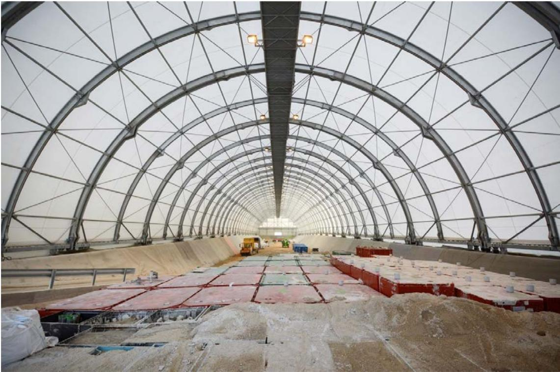
FIG. 18. Premorail shelter over the filled trench of CIRES facility (courtesy of Andra).
