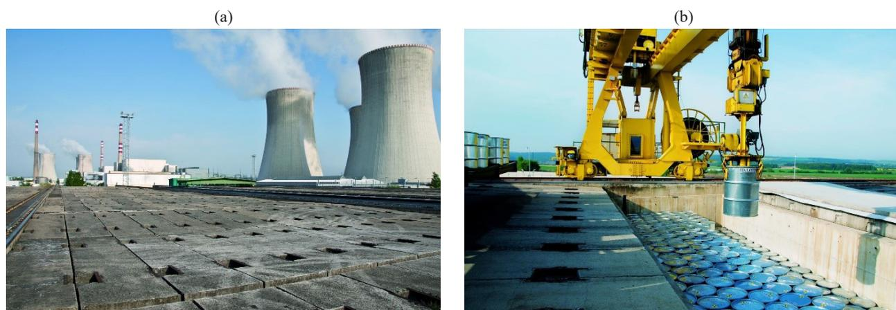
FIG. 25. Dukovany Repository, Czech Republic. Temporarily covered disposal chambers (a) prior to waste emplacement and (b) during waste emplacement activities (courtesy of SÚRAO).
