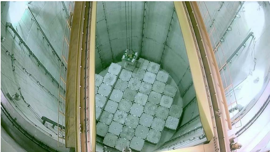
FIG. 31. Waste emplacement operations in a silo at the Wolsong Low- and Intermediate-Level Radioactive Waste Disposal Centre, Republic of Korea (courtesy of KORAD).
