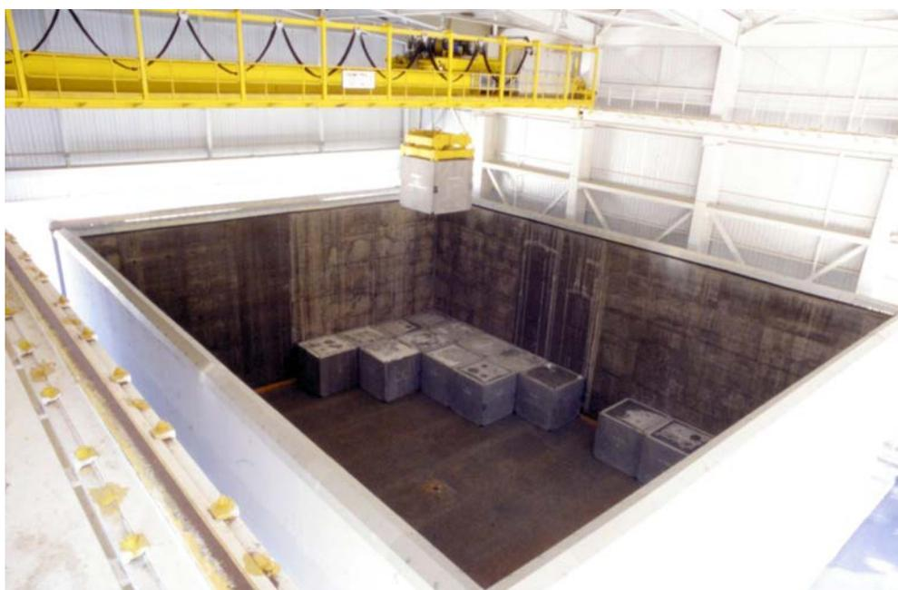
FIG. 23. Filling a vault at the El Cabril LLW repository (courtesy of Enresa).
