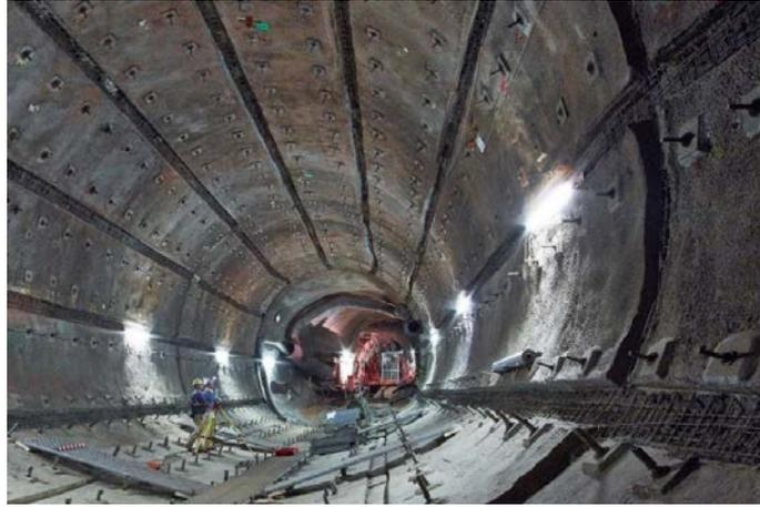
FIG. 48. Construction of a transport drift at the Konrad repository, Germany (courtesy of Bundesgesellschaft für Endlagerung mbH).
