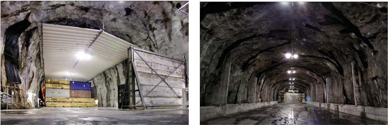
FIG. 33. Disposal vaults for LLW at the SFR, Sweden (courtesy of SKB).
