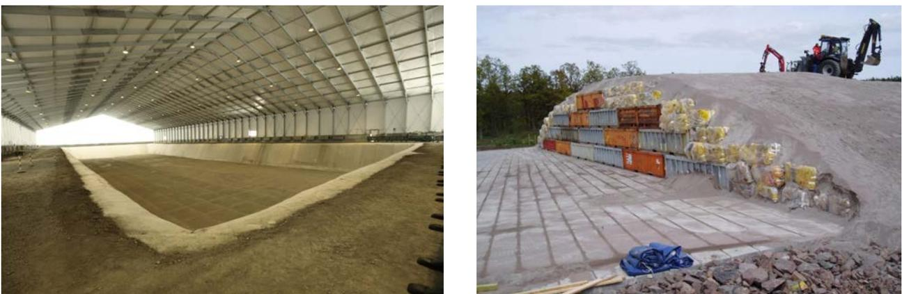
FIG. 16. VLLW disposal: trench at El Cabril, Spain (courtesy of Enresa) (left) and mound at Oskarshamn Nuclear Power Plant, Sweden (courtesy of Svensk Kärnbränslehantering) (right).
