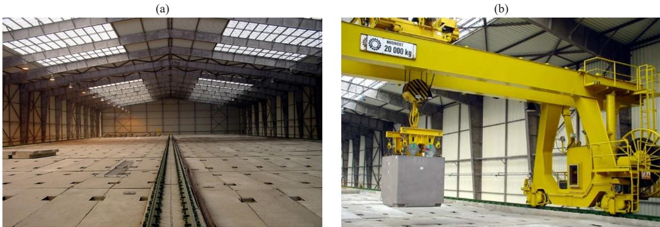
FIG. 27. Mochovce Repository, Slovakia. (a) Covered disposal system with chambers protected by concrete panels and (b) waste package being moved for disposal (courtesy of JAVYS, Slovakia).
