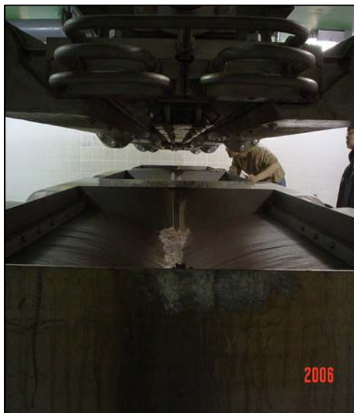
Window is open to wastewater
