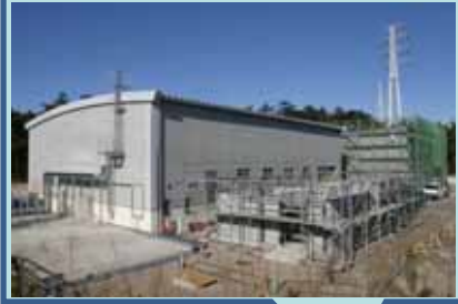
Neutrino monitor building
