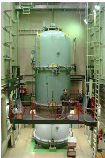
FIG.10. Pelletron-6 accelerator-based system.
