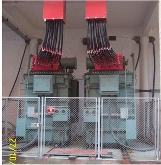
Fig. 7, Multisecondary transformers.
