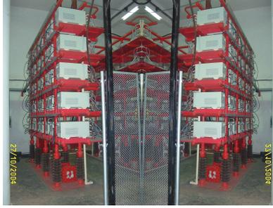
Fig. 6, RHVPS with switched power modules in rack.
