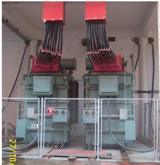
Fig. 7, Multisecondary transformers.
