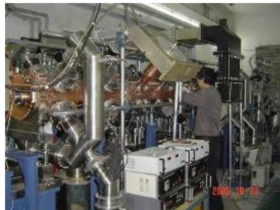
FIG.4 The ADS RFQ installed at IHEP.
