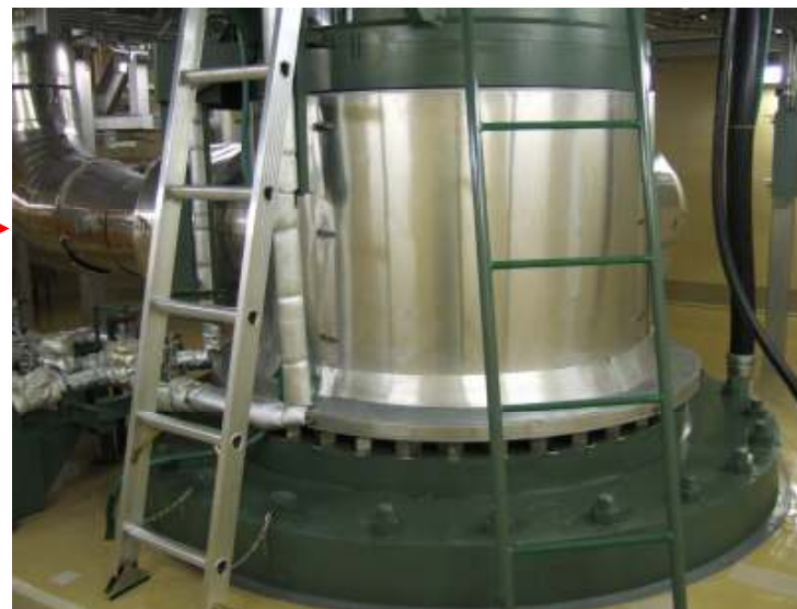
RHR pump (B5F in the reactor building).
